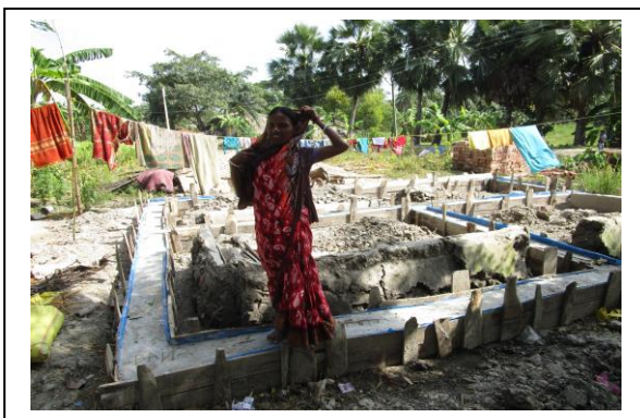
Naratom Pal has started his new house supported by the Government.
